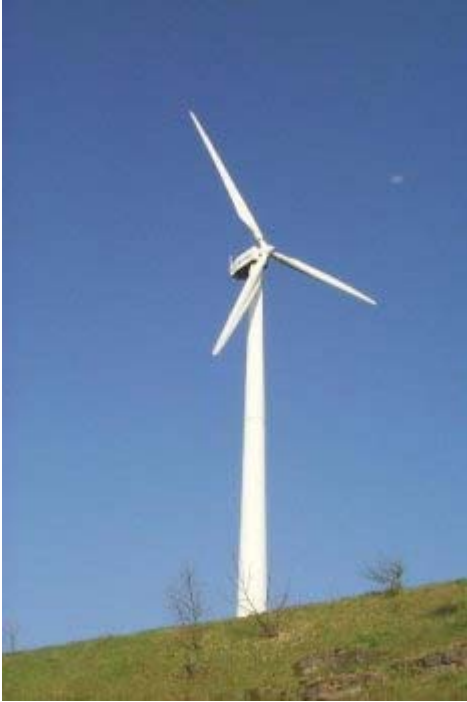
This is the 100-kilowatt-capacity Fuhrländer wind turbine model planned for the Luna Point project. (Photo courtesy of Lorax Energy Systems/ Northwest SEED)
