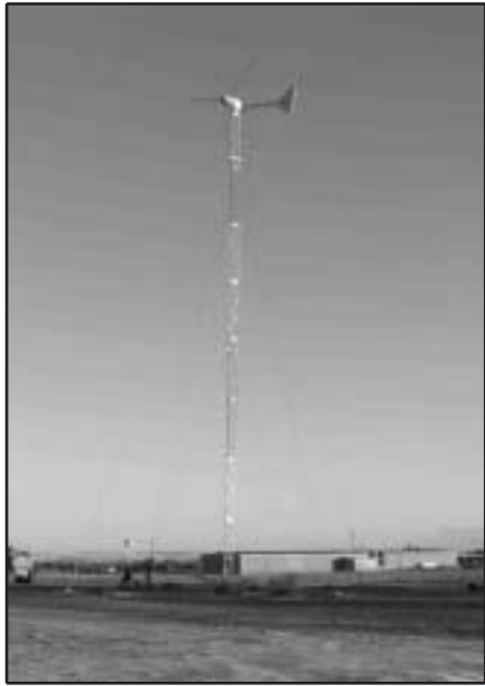
Liberty County's newly built 10 kW, the third Montana turbine installed as part of Our Wind Co-op. Photo credit: Don Marble
