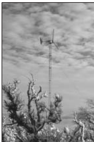
Ed Kennell's 10kW Bergey atop the wintry Luna Butte. Photo Credit: Ed Kennell.
