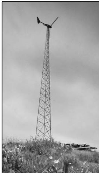
Don and Beverly Grim's 10 kW turbine in Peshastin, WA
