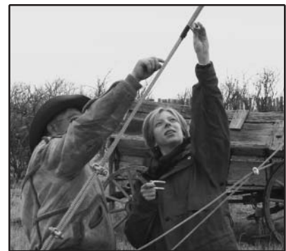
Sarah Peterson places guy wire clamps on Jess Alger's turbine in Stanford, MT
